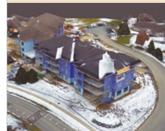
Aerial view of Pheasant Pointe while under construction earlier this year.
